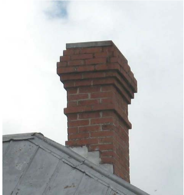
The distinctive corbelled brick chimney at 600 Adams Street should be reconstructed to match its historic appearance if it needs extensive repairs or replacement.
