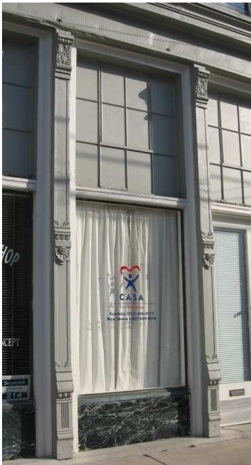
The painted finish of these cast iron columns at 212 Willow Street helps to protect them.
