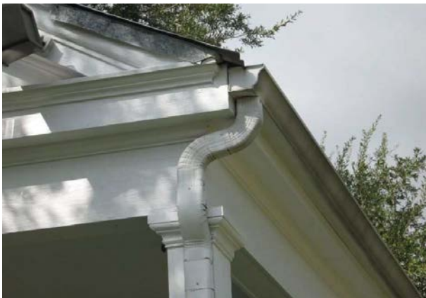
The downspout on 301 Iberia Street uses placement at a corner and coloring that matches its adjoining surface to minimize its visual effect.
