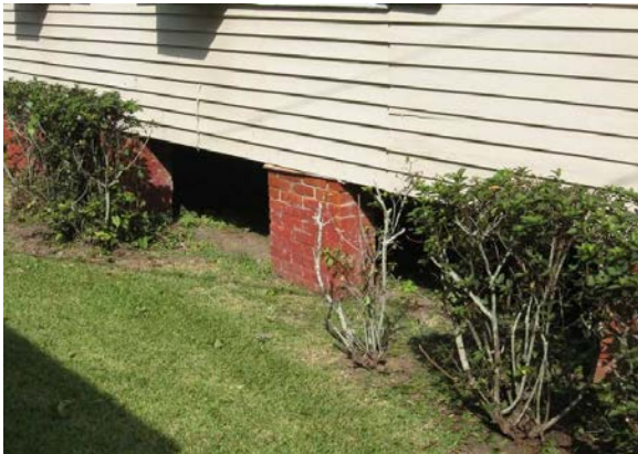
The brick pier foundation of the house at 807 2nd Street has been appropriately left uncovered.
