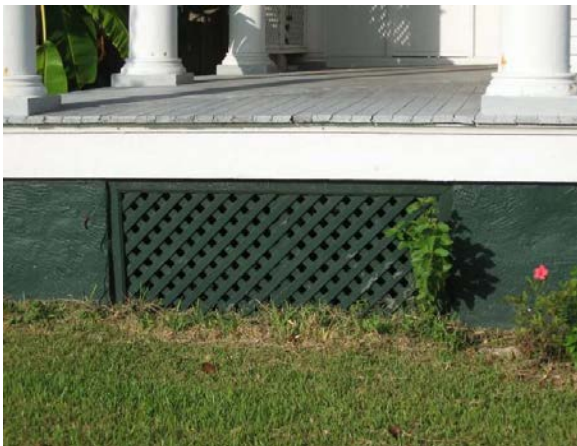
The pier foundation at 817 Main Street has appropriately been left visible, with lattice inserted in between piers, rather than covering them.
